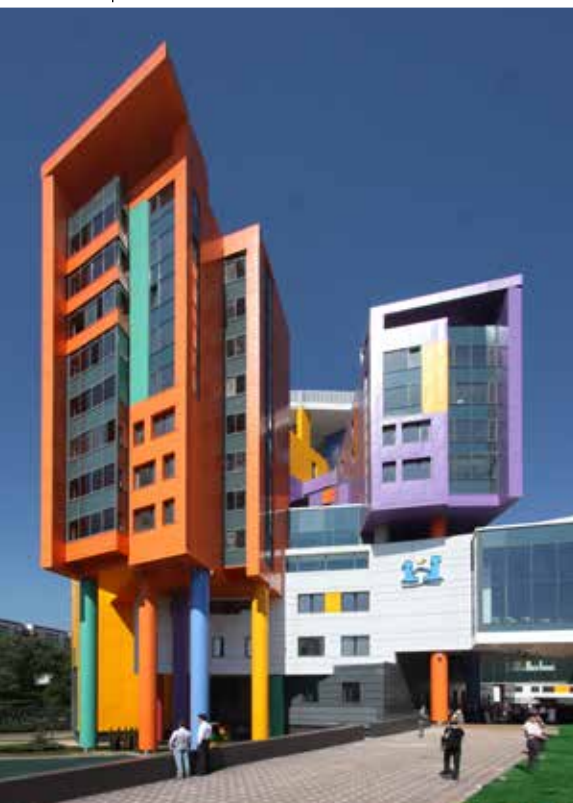
Moscow hospital – Moscow, Russia Moscow project institute & asadov architectural studio Prepainted metal sheets: Novelis
