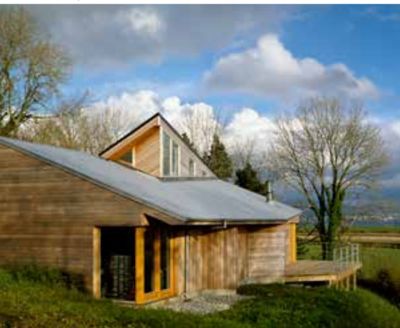
Carton Levert house – County Donegal, Ireland Macgabhan architects Prepainted metal sheets: Tata Steel
